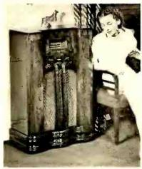
Seven-tube two-band receiver with trimmer push-button tuning, magic eye, straight line dial and metal tubes. Console cabinet—two bands, 530-1720 and 2300-22,000 KC, covering domestic and foreign broadcast. Has 4.5 watts output, 12" dynamic speaker, 20 to 1 vernier tuning, phono-connection, AVC, wave trap, automatic tone compensation and iron core I.F. transformers. Lists at \$89.95. RCA Mfg. Co., Camden, N. J—RADIO TODAY—see also advt. page 21.
